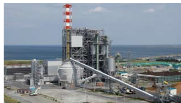
Overall view of the biomass power generation plant
